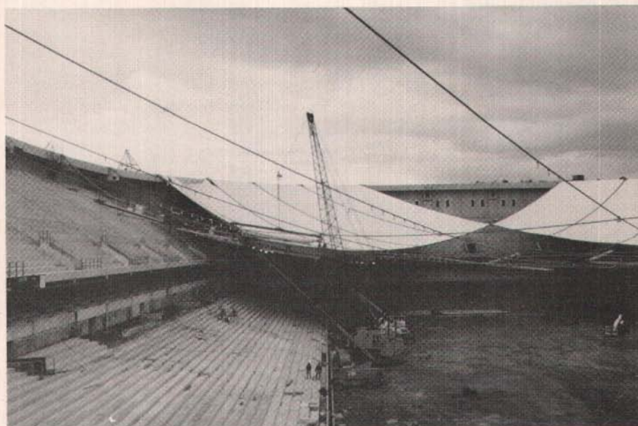
Erection of the roof fabric over the strung roof cables. The gig supported by an overhead cable spools out the fabric roof panels which are clamped to the roof cables.
