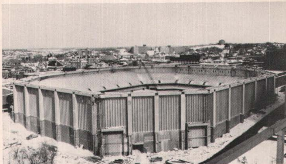
The erected stadium bowl 8 months after ground was broken. The precast double tees and columns create a clean and maintenance free exterior.
