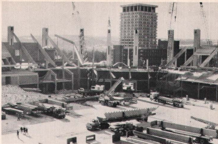
Construction of the stadium bowl. The interior arena space lends itself readily for storing the precast columns and bents.
