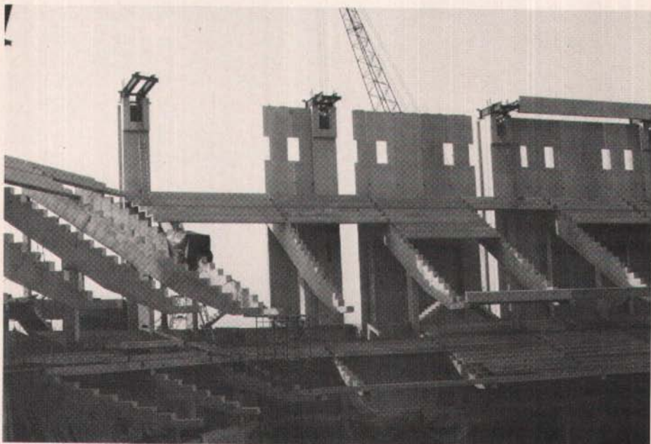
Erection of the exterior wall system. Openings in the wall panels are for air intake dampers. Note the cantilevered steel dunnage to receive the inside precast flange for the "U" shaped ring beam.
