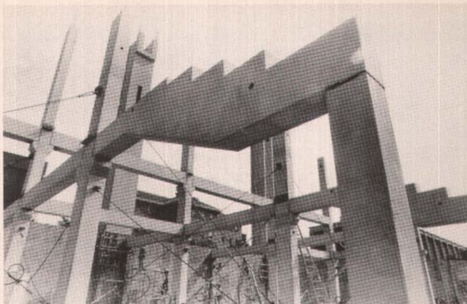
Precast prestressed concrete frame in place.
